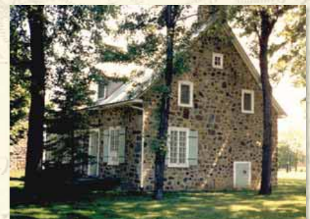
Foundation House, Sisters of the Holy Names Longueuil, Quebec, constructed circa 1740
